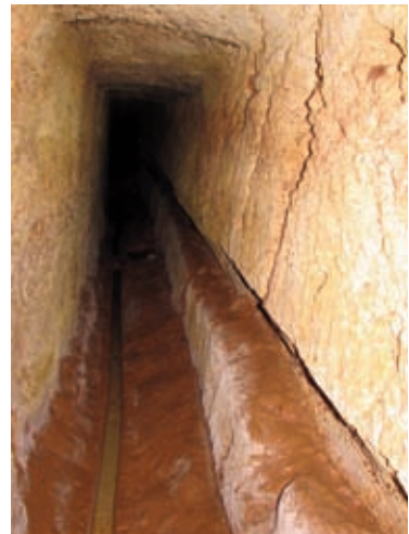
Fig. 10.8. Canals are often carved into the floors of galleries in order to ease the water flow retrieved from the perched aquifer.
